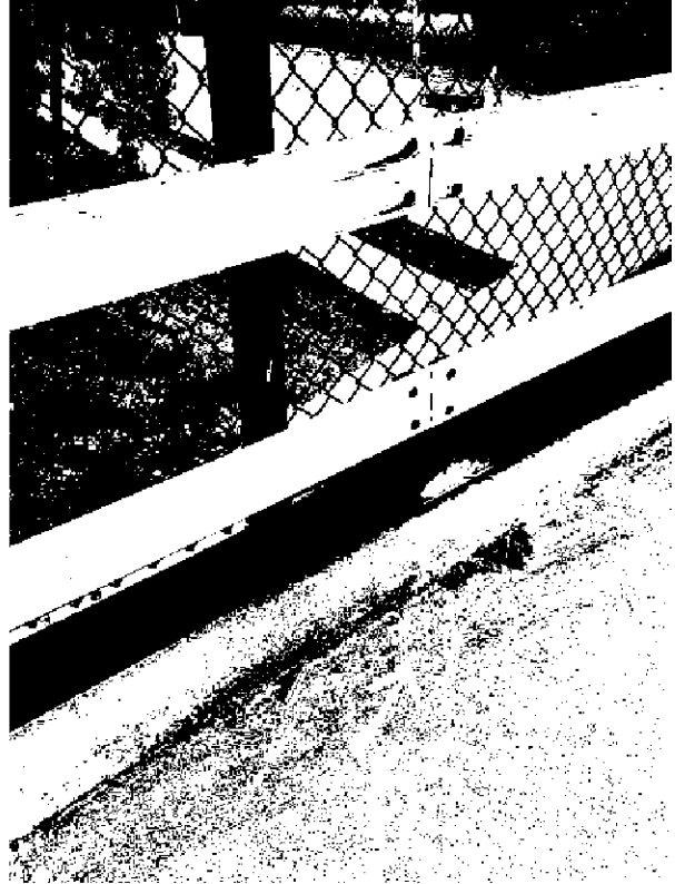
Deformed fence post at 155' from northeast abutment.
