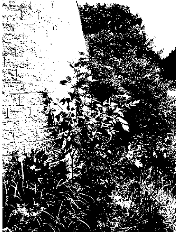
Significant woody plant growth along the northeast abutment.
