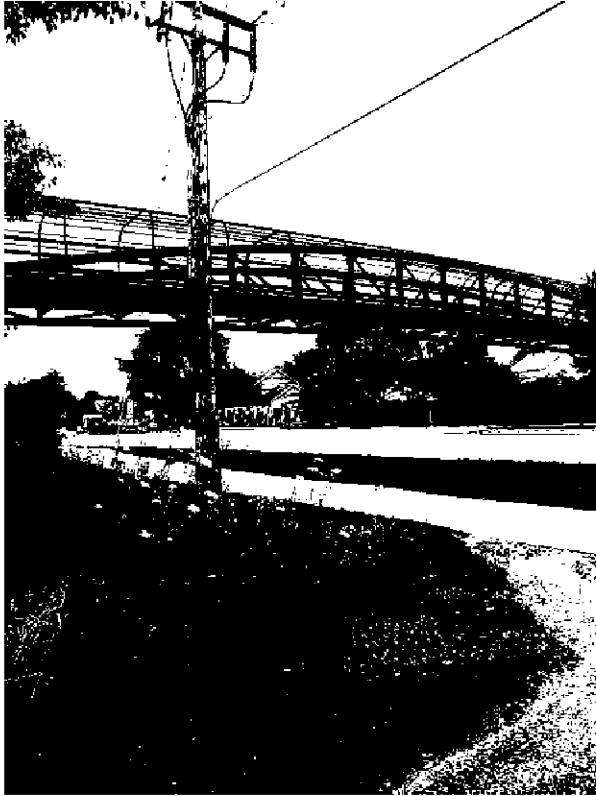
Southeast side of structure.
